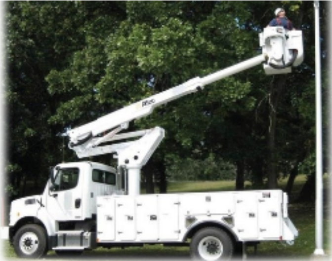
Aerial Cable Placement (Bucket Truck)
