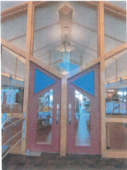
Interior front doors
