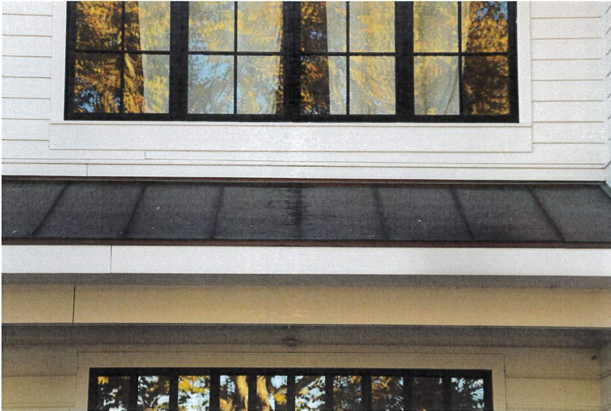
EXAMPLE OF COPPER ROOF
