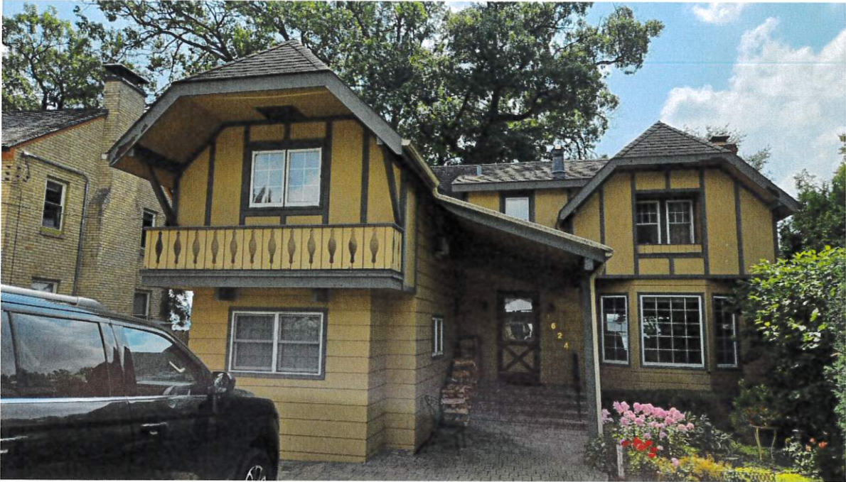
View from Street (West looking East)
