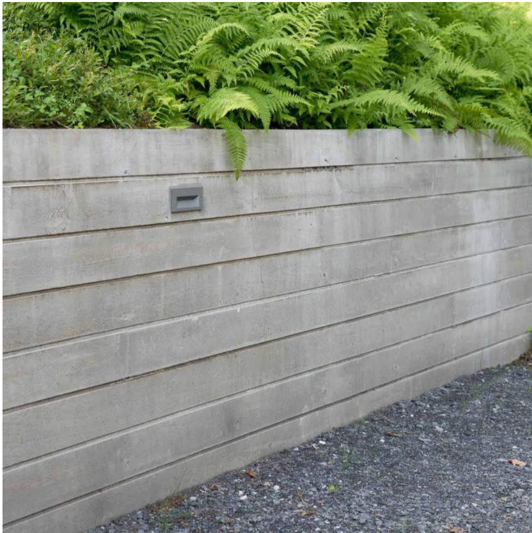
CONCRETE - BOARD FORM
