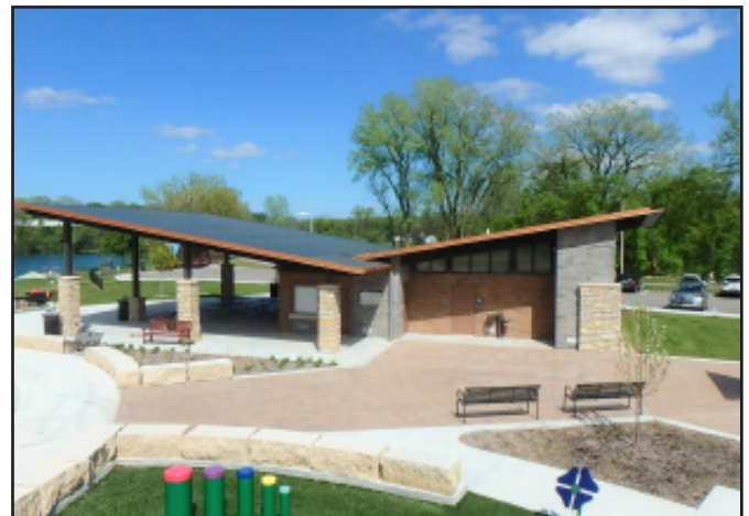
Park Shelter and Restroom - Verona, WI
