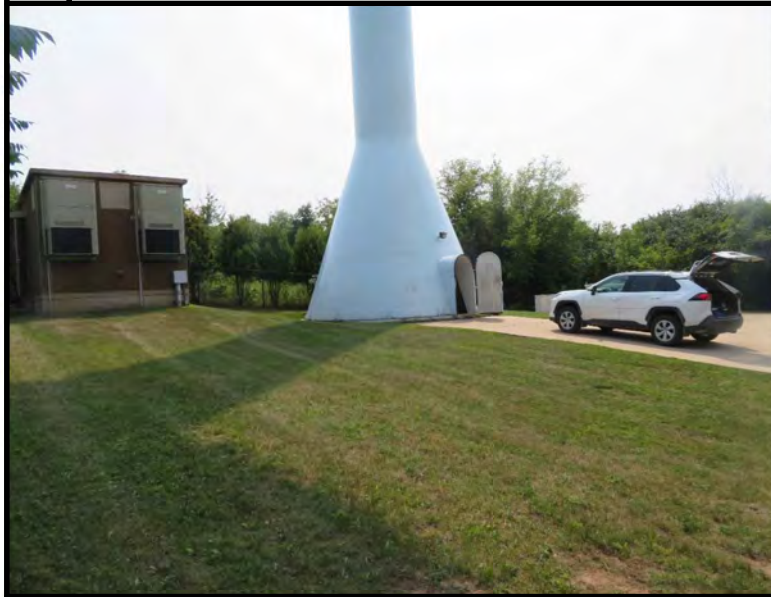
B COMPOUND OVERVIEW
