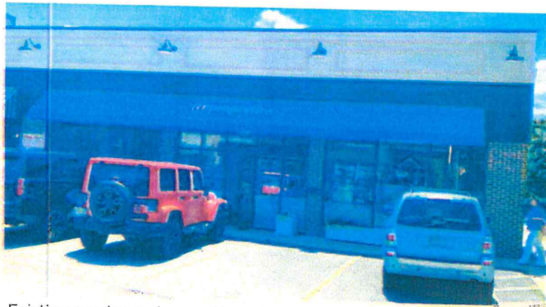
Existing awning to be re-skinned
