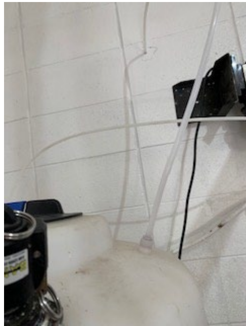
Wellhouse #4 Sodium Hypochlorite Venting
