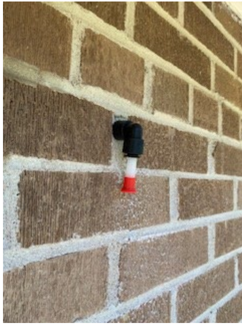
Wellhouse #3 Sodium Hypochlorite Venting
