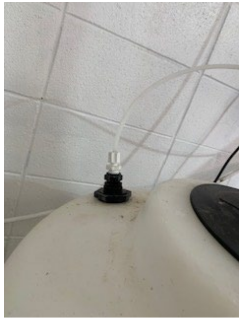
Wellhouse #5 Sodium Hypochlorite Venting
