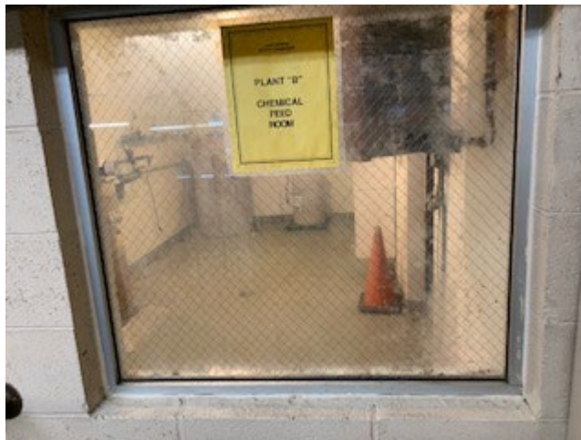
Plant B Chemical Room Window
