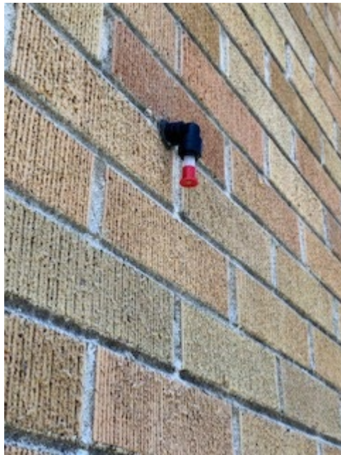
Wellhouse #4 Sodium Hypochlorite Venting
