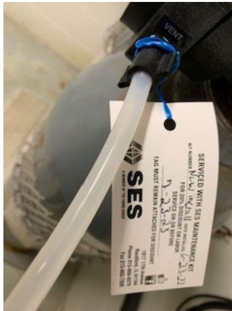
Plant A Fluoride and Chlorine Gas Venting
