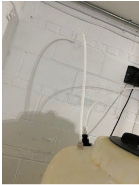
Wellhouse #3 Sodium Hypochlorite Venting
