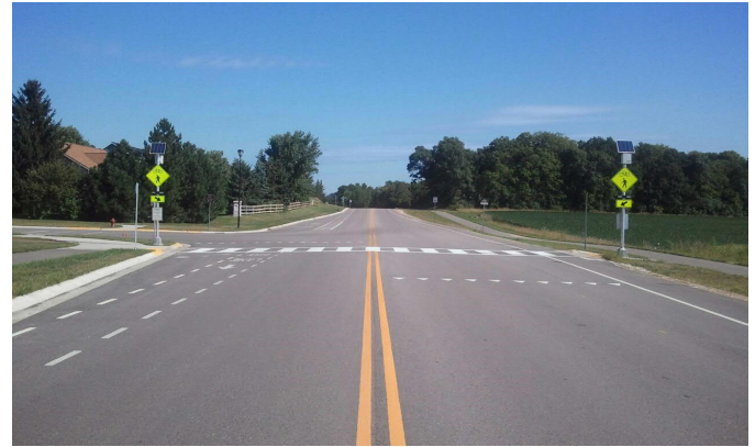
Pedestrian crossing on Woodland Drive in Waunakee, Wisconsin, including rectangular rapid-flashing beacons (RRFB).
