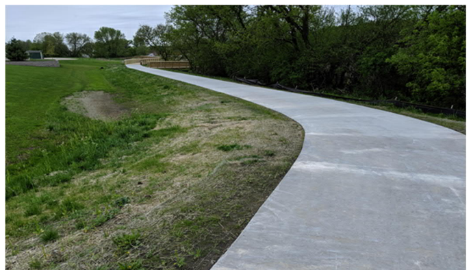
New concrete pavement and wooden boardwalk trail provided pedestrian connectivity by coordinating with multiple entities.
