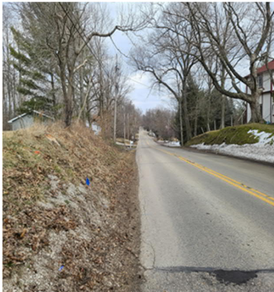
Existing grade changes between the roadway and trail alignment may require retaining walls or variances by WisDOT.
