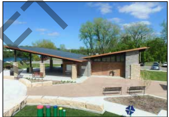
Park Shelter and Restroom - Verona, WI
