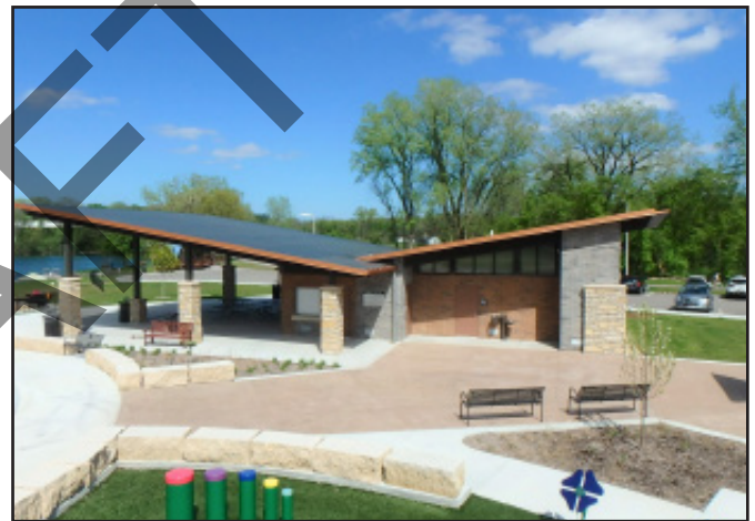
Park Shelter and Restroom - Verona, WI
