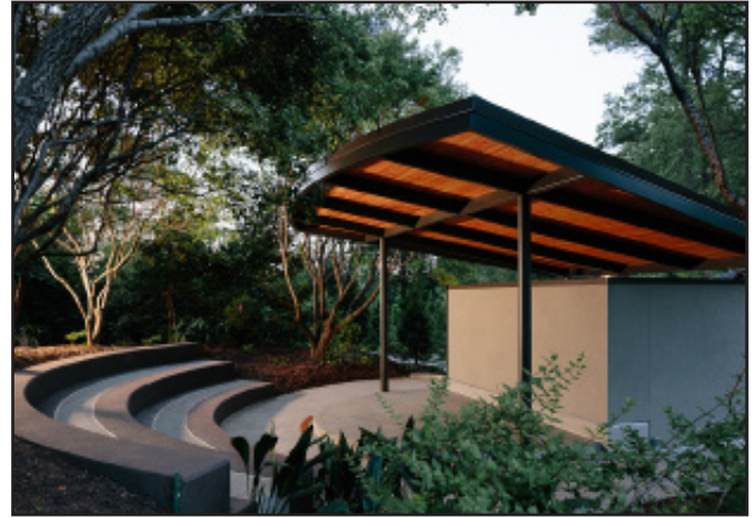
Amphitheater and Restroom - Verona, WI
