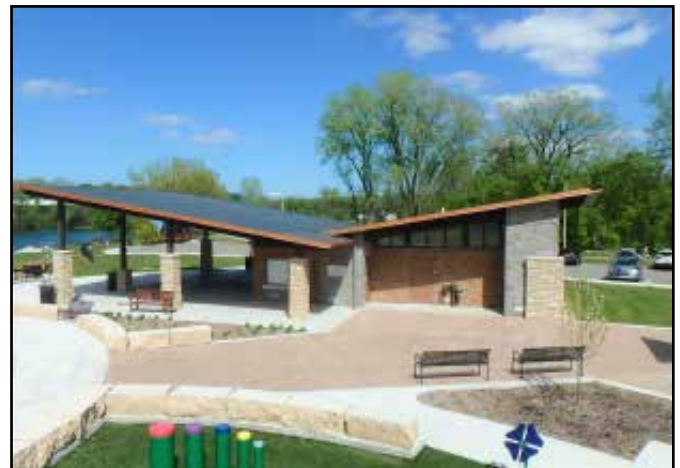
Park Shelter and Restroom - Verona, WI
