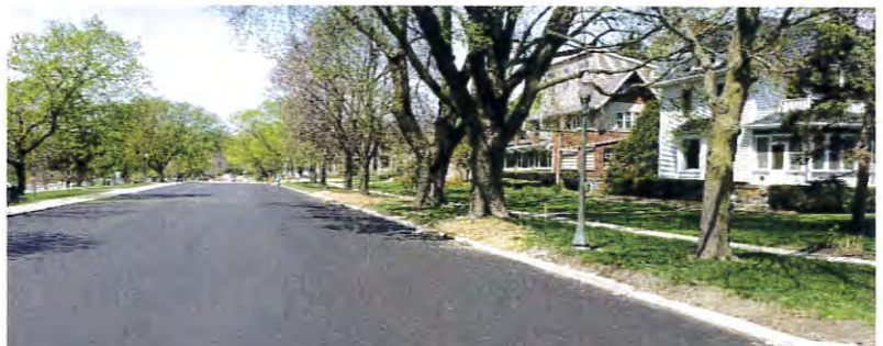
Kapur provides reconstruction and rehabilitation of streets throughout Southeast Wisconsin
