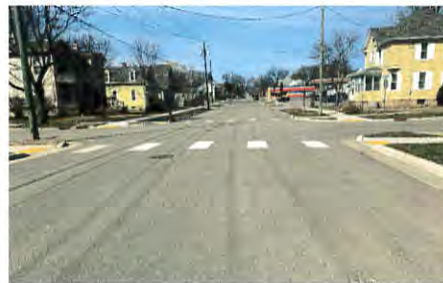
Finished project looking south along Monroe Street – new ADA compliant ramps.
