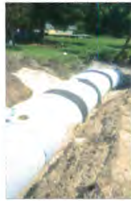
At left, upsized elliptical storm sewer to mitigate flooding. At right, finished street improvements.
