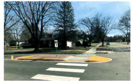
Pedestrian refuge island at ADA compliant crossing.
