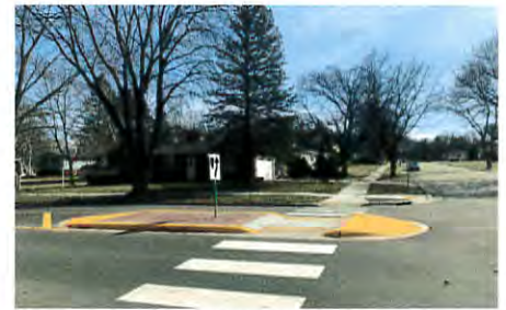
Pedestrian refuge island at ADA compliant crossing.
