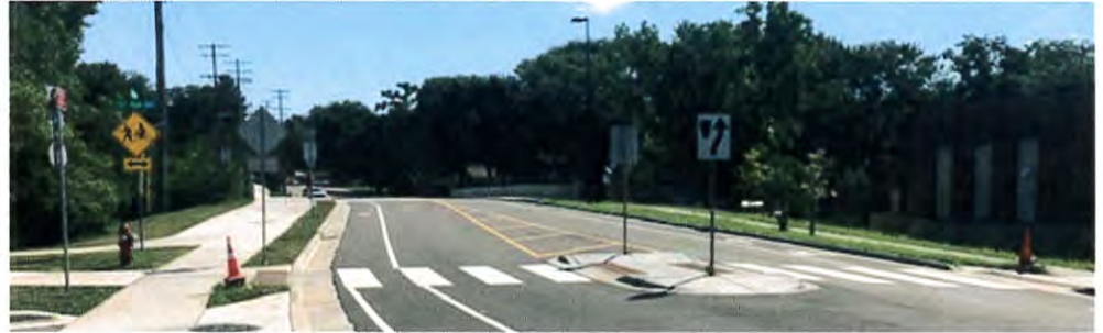
Finished project with pedestrian refuge island and ADA compliant sidewalk improvements.
