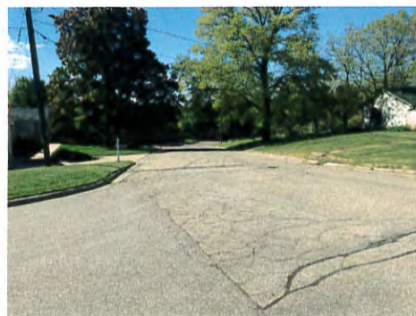
Sky Lane Drive existing pavement.
