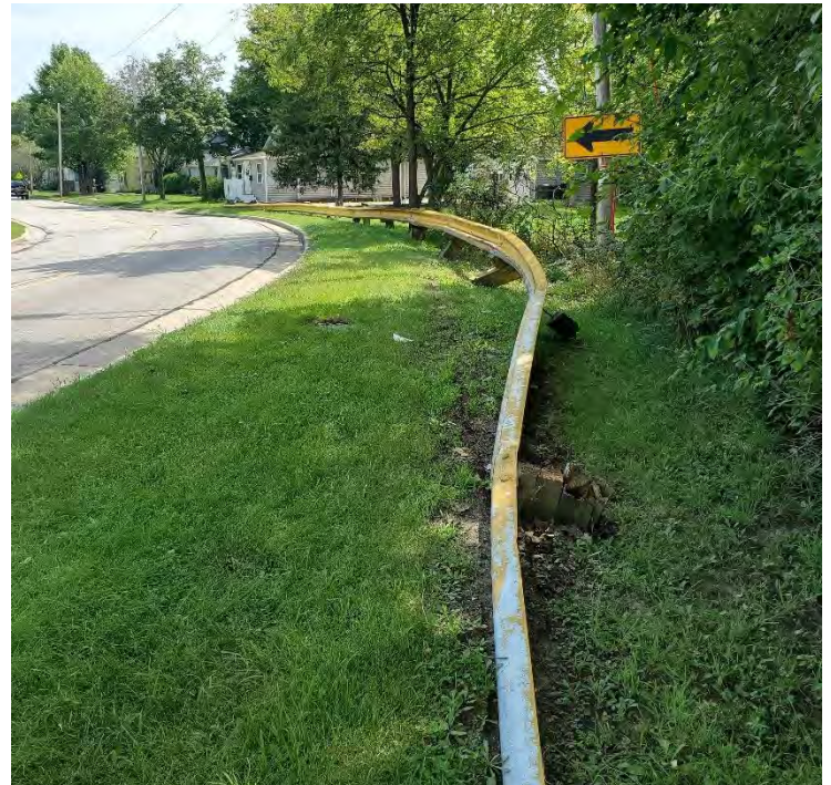
Figure 3: Existing Guardrail on George St.
