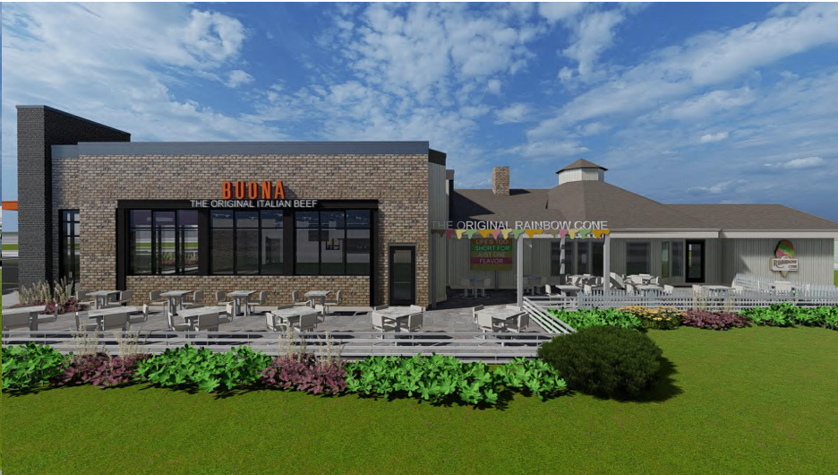
SOUTH SIDE, FACING MAIN ROAD
