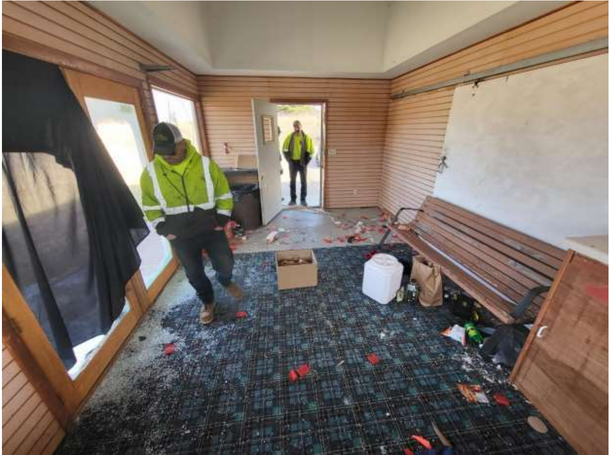
Driving Range Office on Hillmoor Property:
