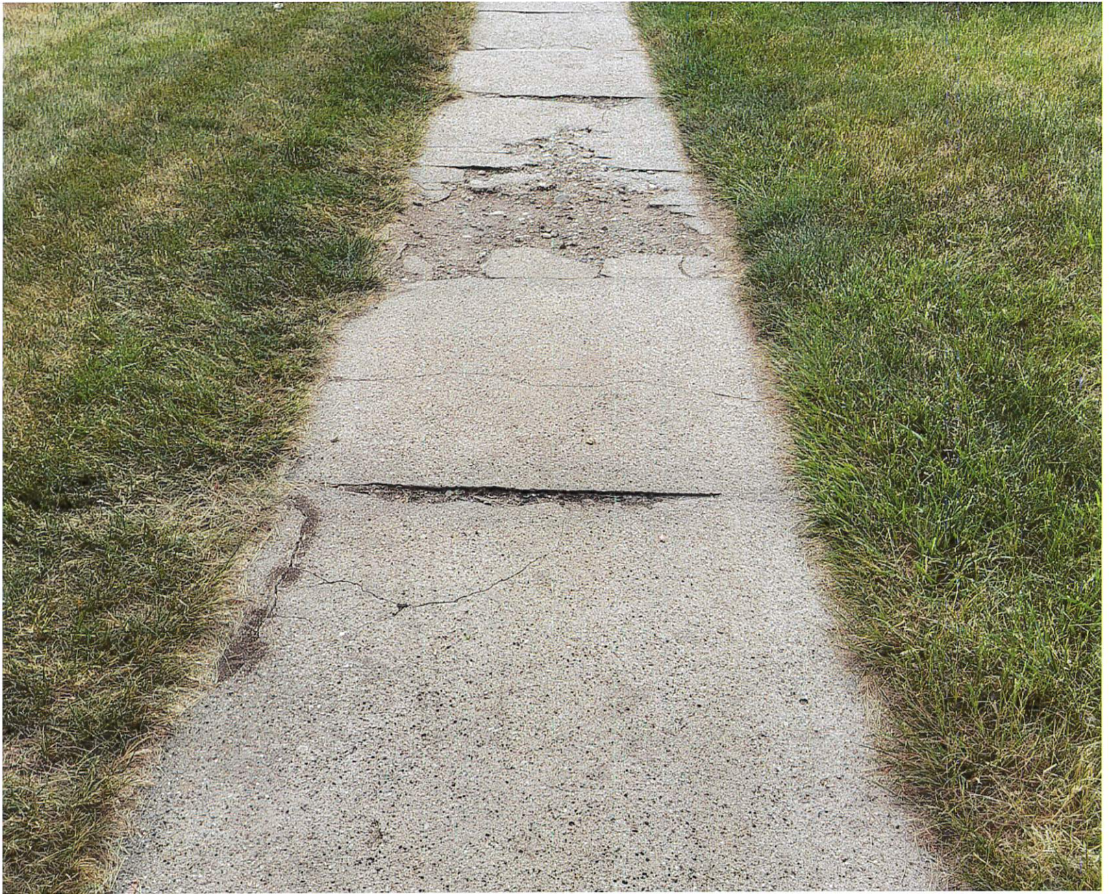
Summer Haven Wells St. Frontage (West Side)
