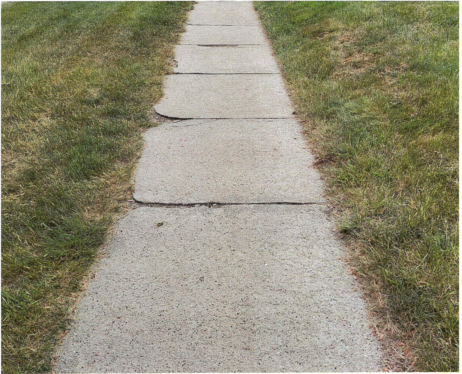
Summer Haven Wells St. Frontage (West Side)
