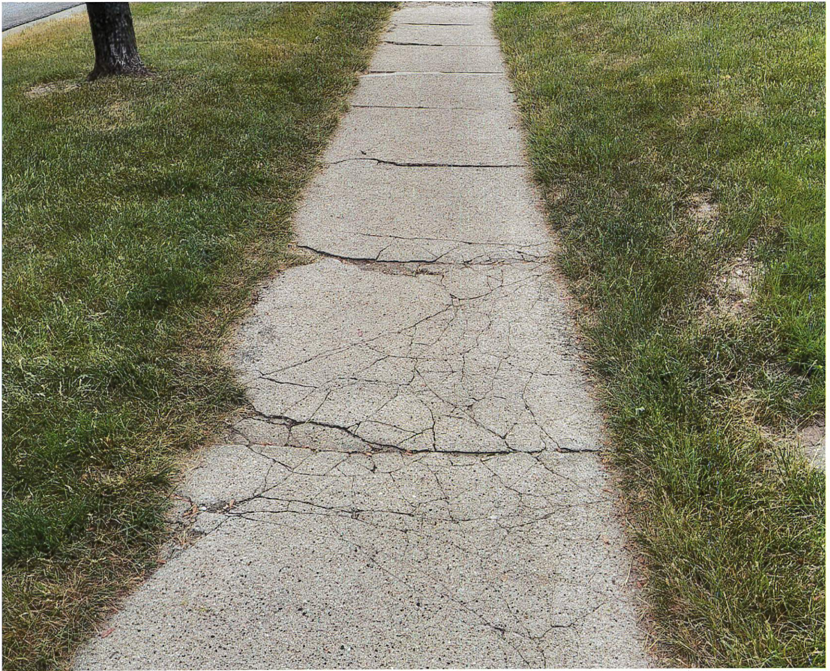
Summer Haven Wells St. Frontage (West Side)
