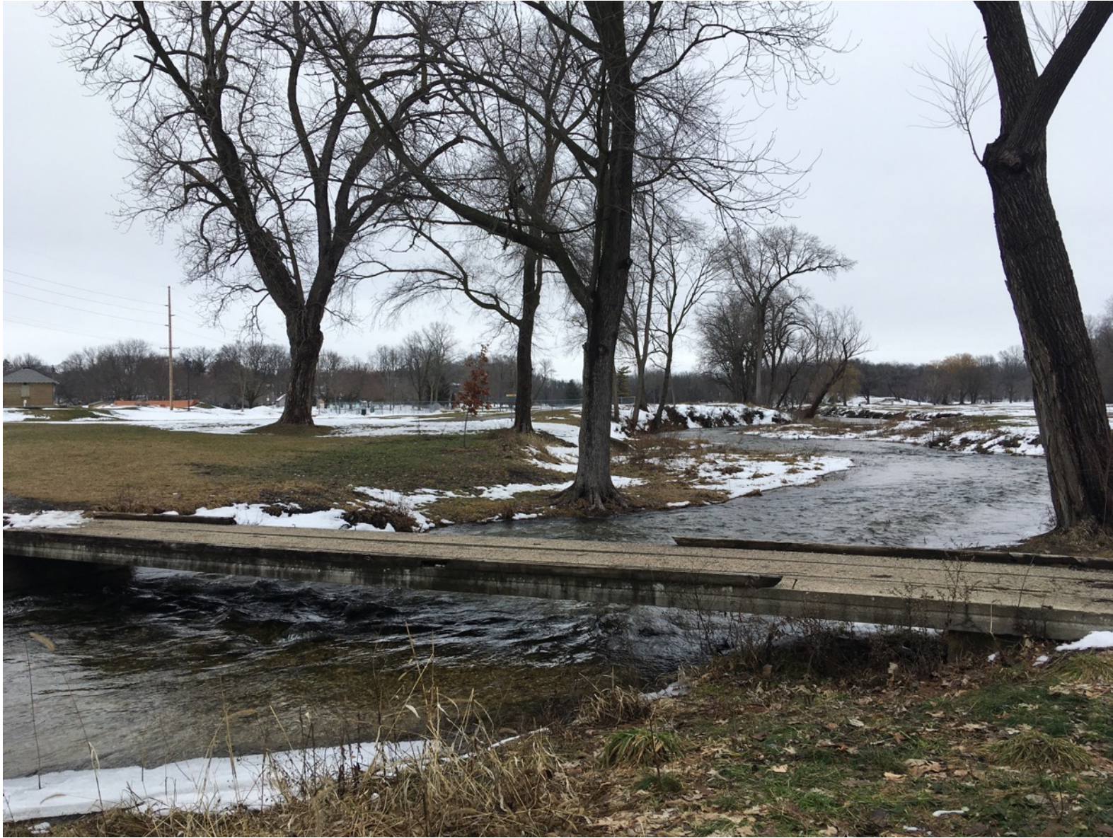
Bridge #5 (cement foot bridge)
