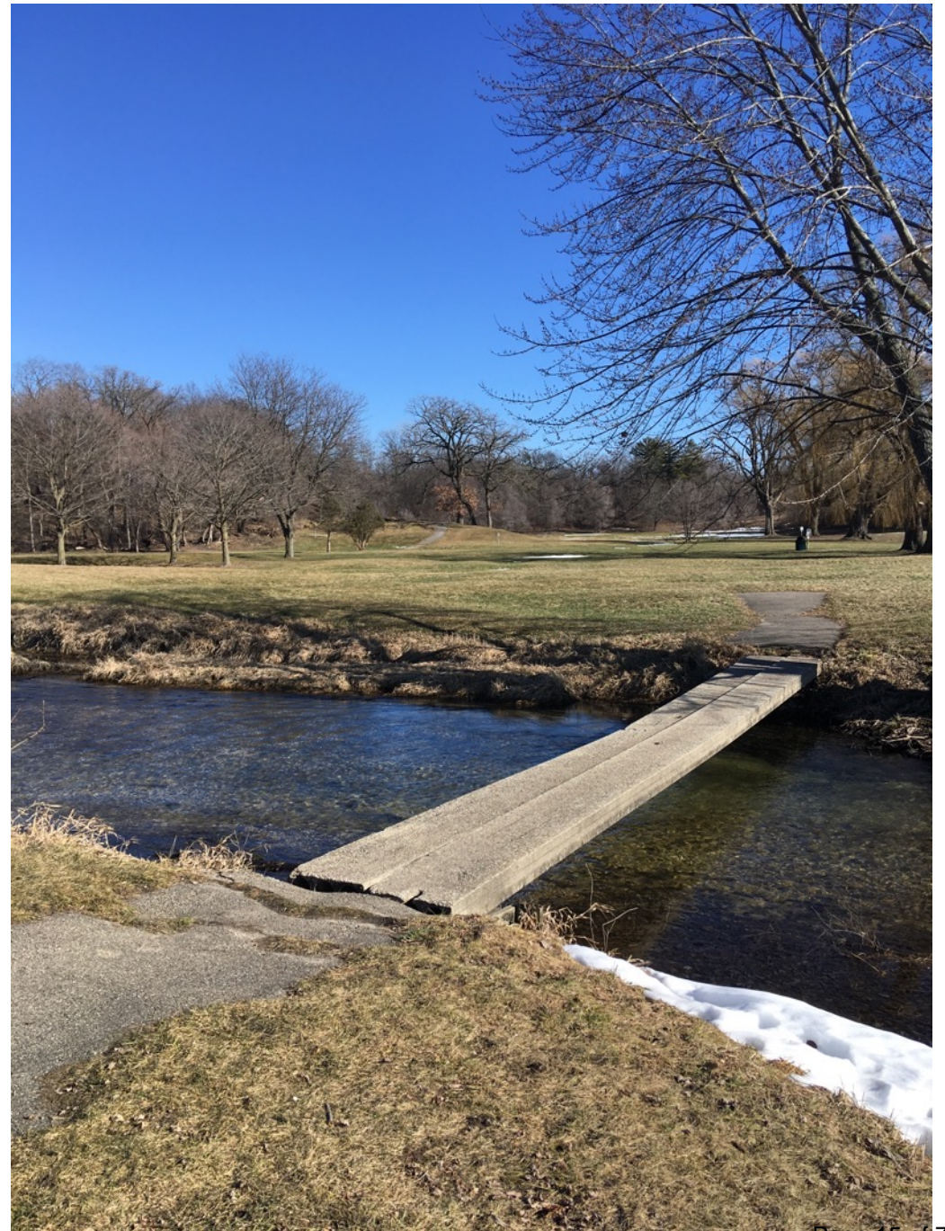
Bridge #2 (to be replaced by City?)
