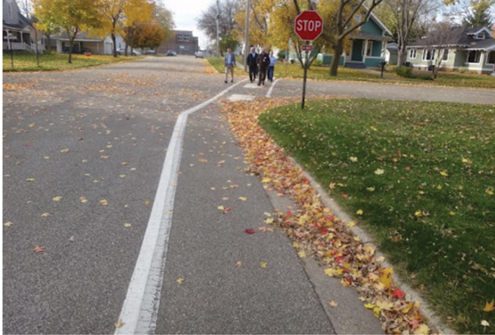
VISUALLY SEPARATED PEDESTRIAN LANE IN ST. CHARLES, MN
