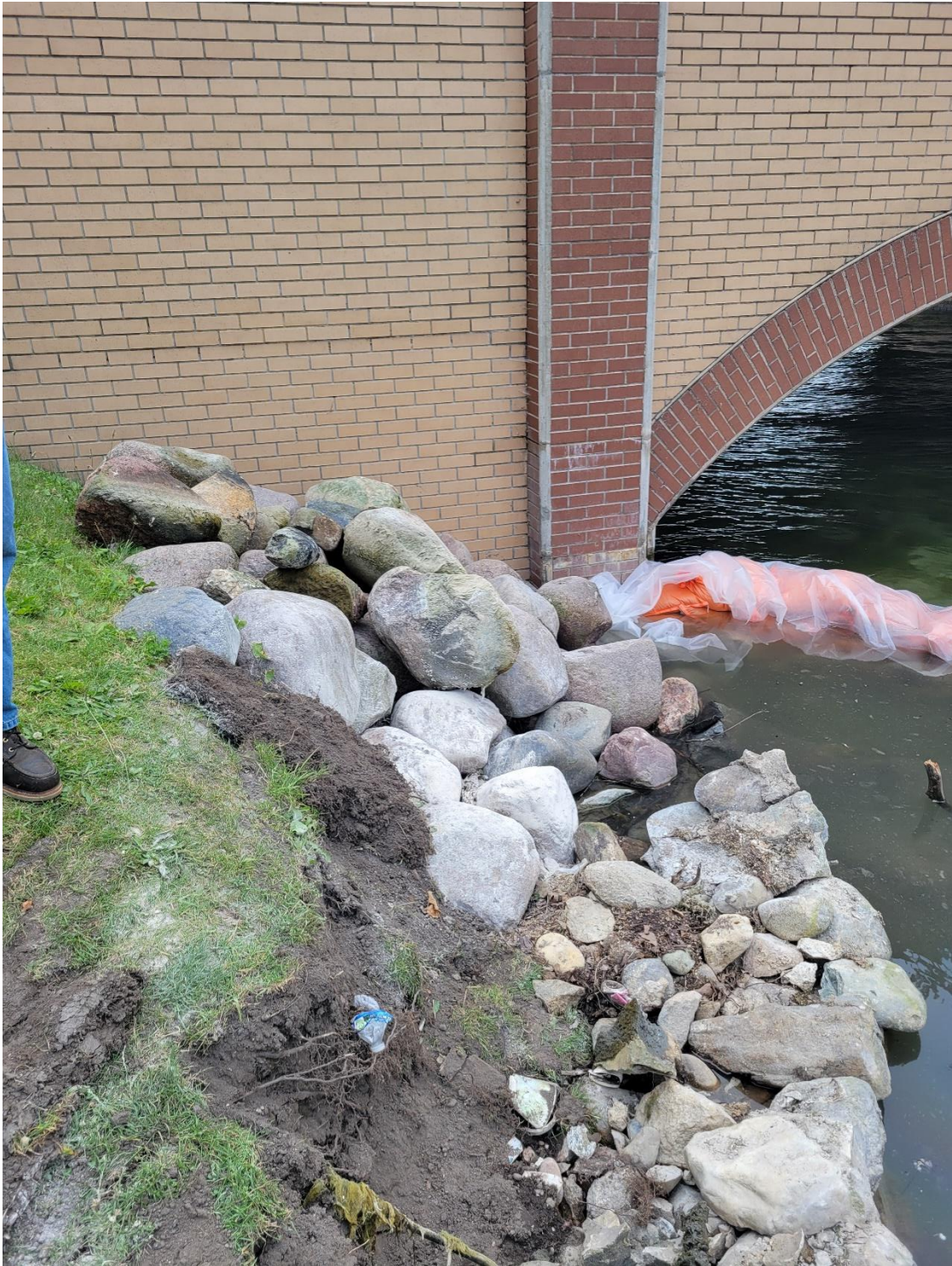
Picture of the Existing Armoring Near the Wrigley Drive Bridge, Facing West
