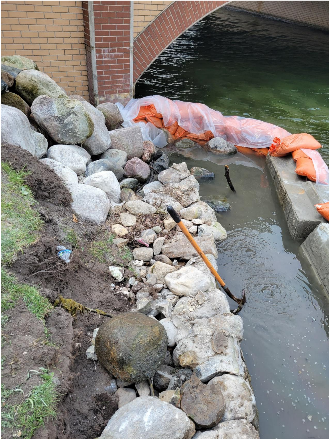
Picture of the Existing Seawall with Concrete Cap Removed, Facing West
