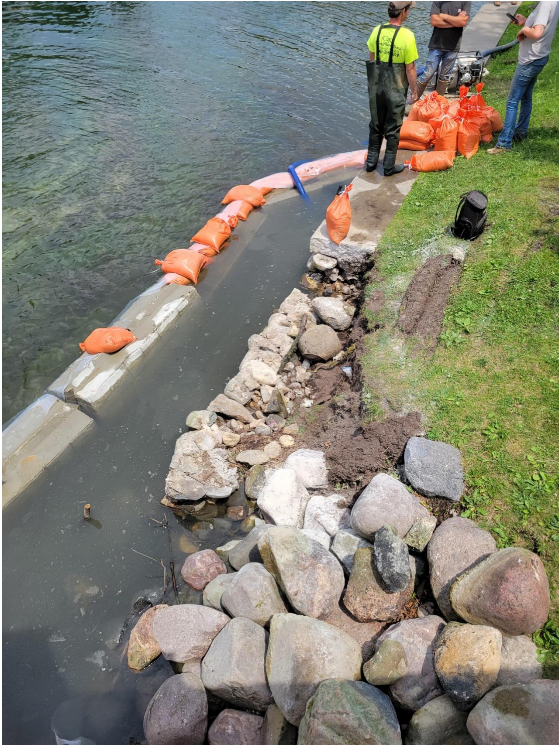
Photo of Existing Armoring and Existing Seawall, Facing East
