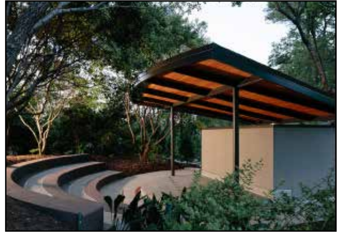
Amphitheater and Restroom - Verona, WI
