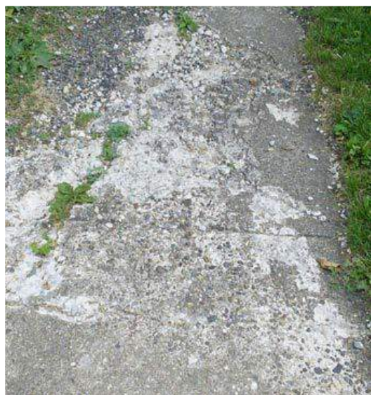
Figure 4: Example of Spalling on a Concrete Sidewalk
