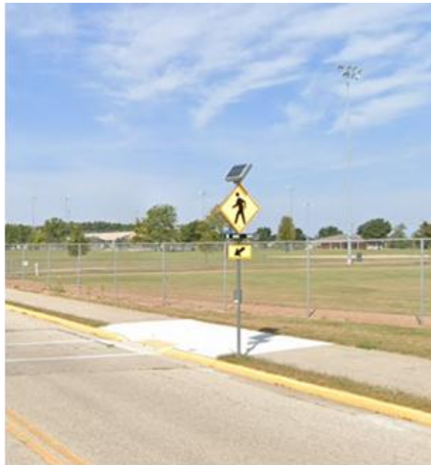
Existing RFB on Townline Rd.
