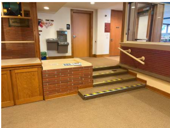
Figure 3 Program Room Stair and Landing
